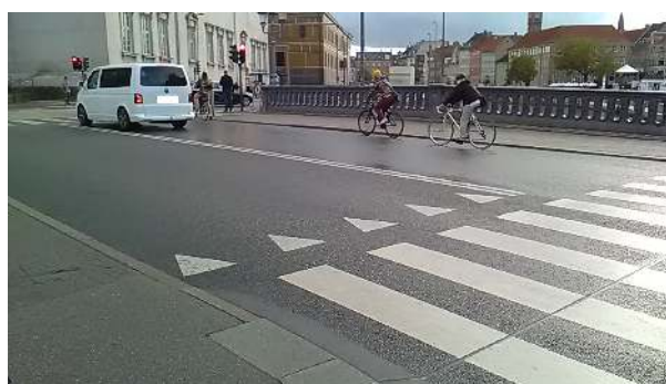
Figure 3.29: Bridge: Gap 66 on Højbro [107]
